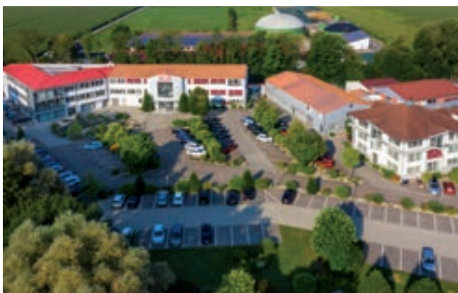
ABUS Security-Center - Augsburg, Germany
